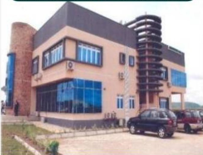
ADMINISTRATIVE BUILDING Accountancy Road, kwall Near Jos, Plateau State
