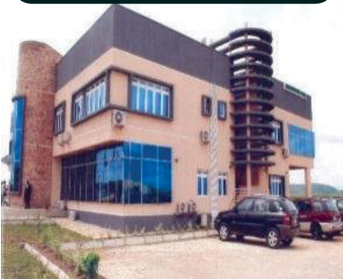
ADMINISTRATIVE BUILDING Accountancy Road, kwall Near Jos, Plateau State
