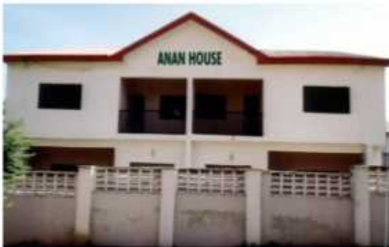
ANAN Annex Office
